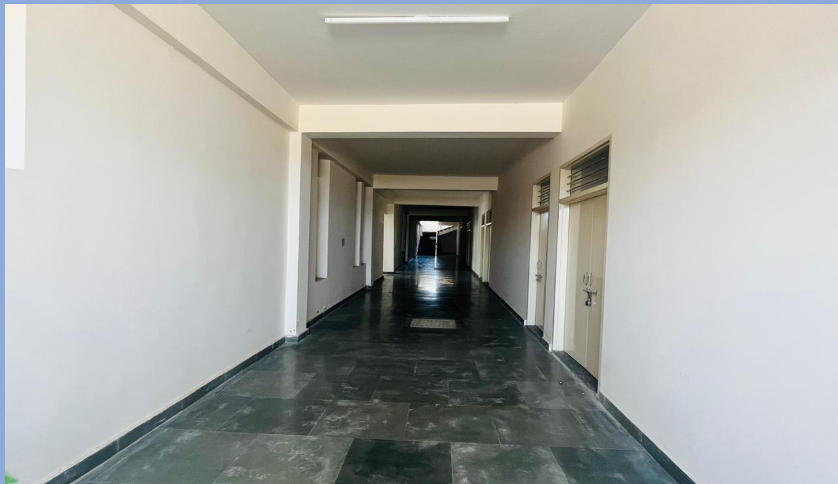
Newly Constructed Extension of A-Block
